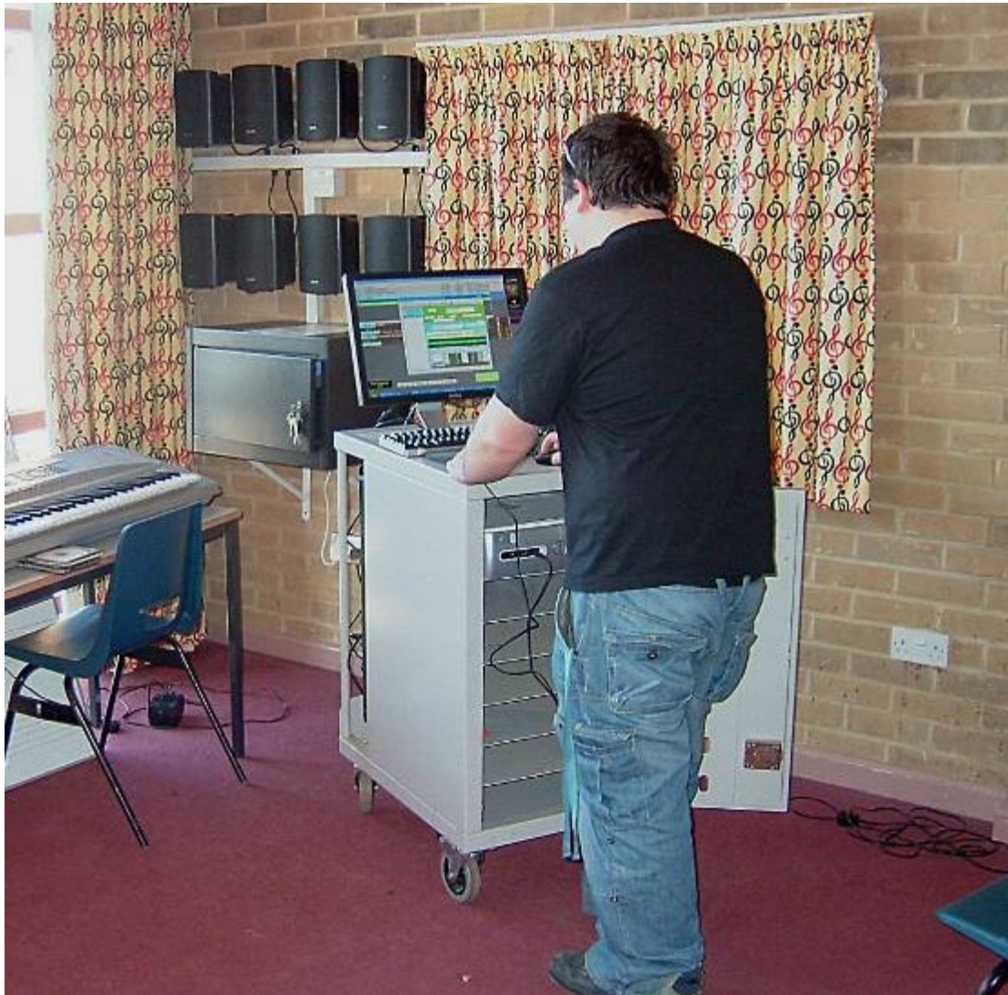
Steve Smith testing the Sound Post equipment after installation
