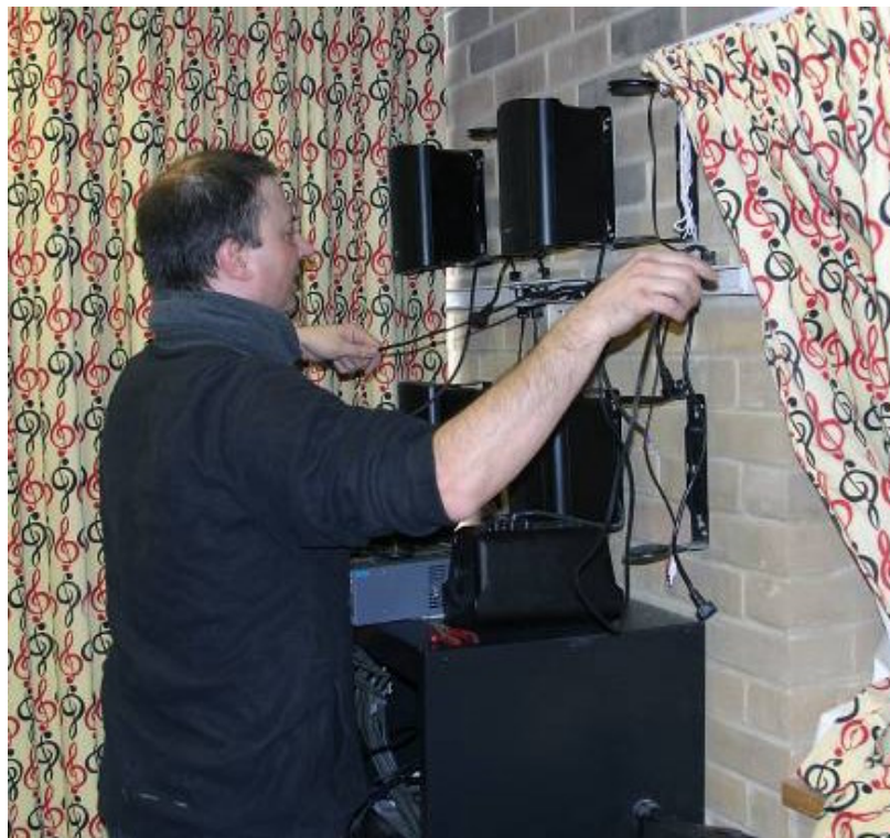
John Boath installing the monitor speakers in the classroom
