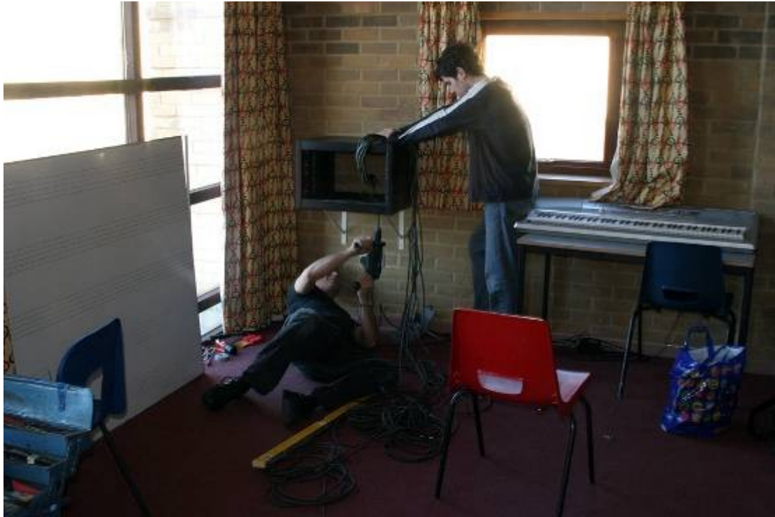
John Boath and Matt Ware working on the classroom installation
